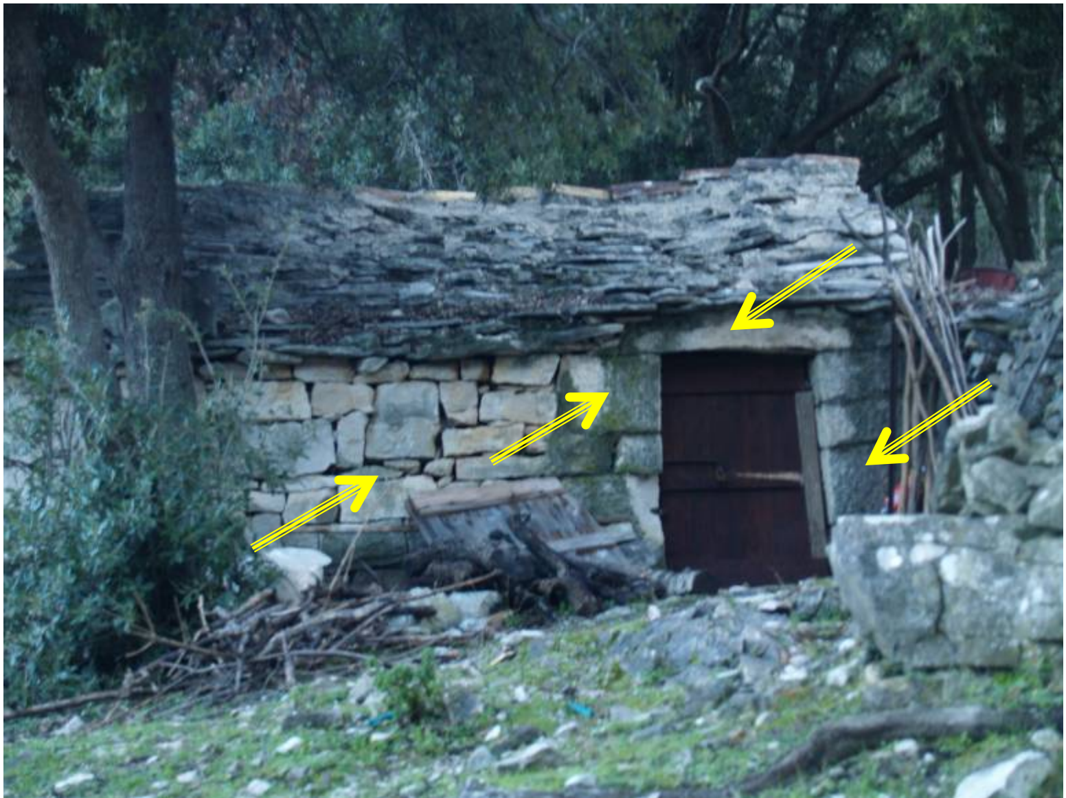
BIG HEADER STONES AT THE CORNERS AND AROUND THE OPENINGS
