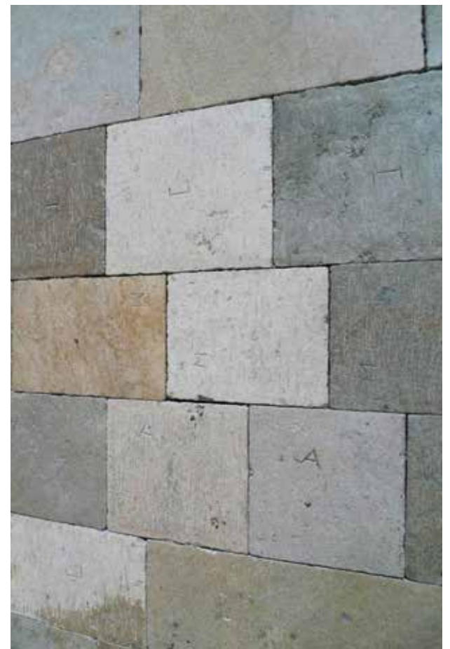
Different traces of stone-cutting tools in the stone
